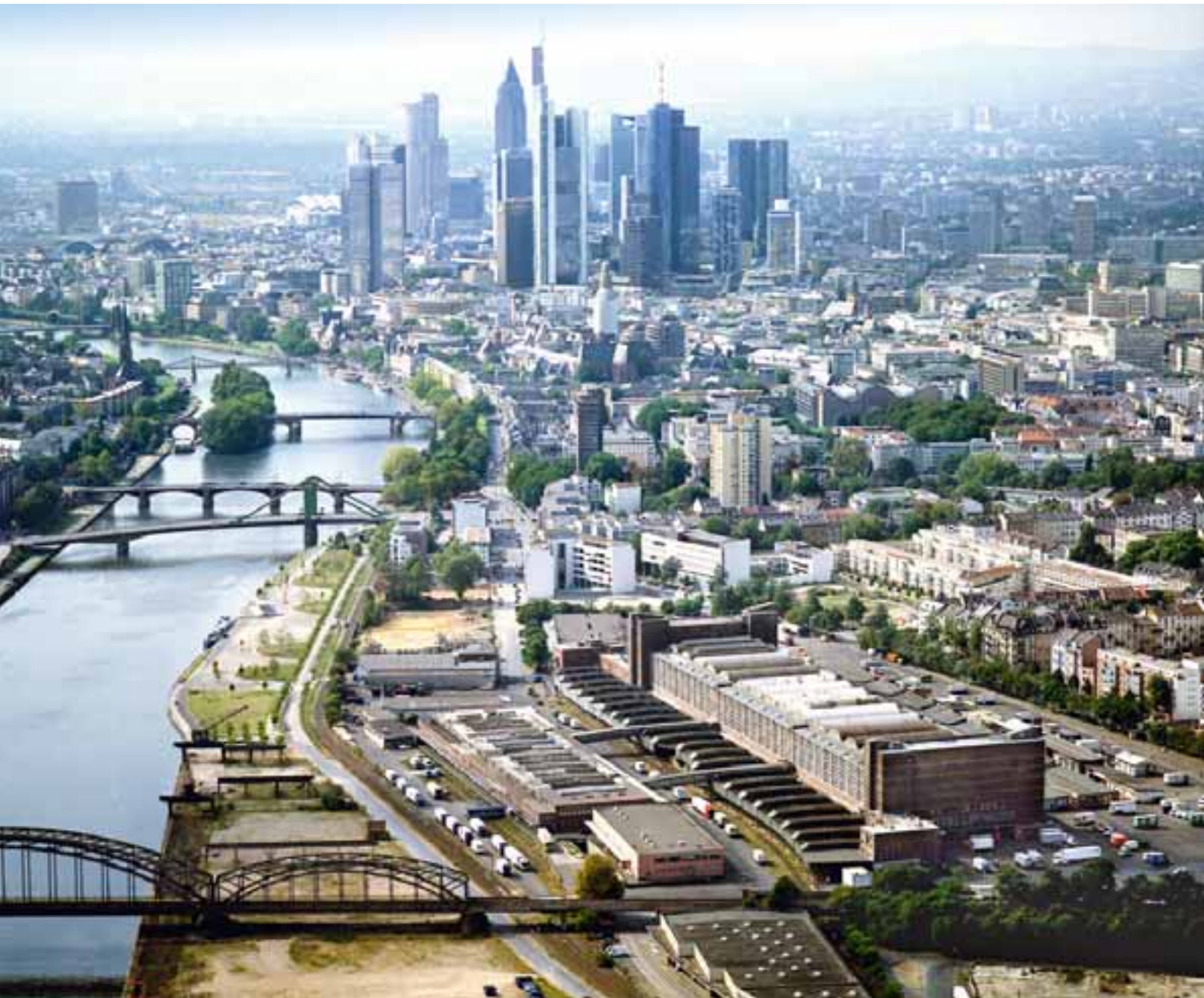
View of the Grossmarkthalle when it was still a wholesale market, with the city centre in the background towards the west (2002).
