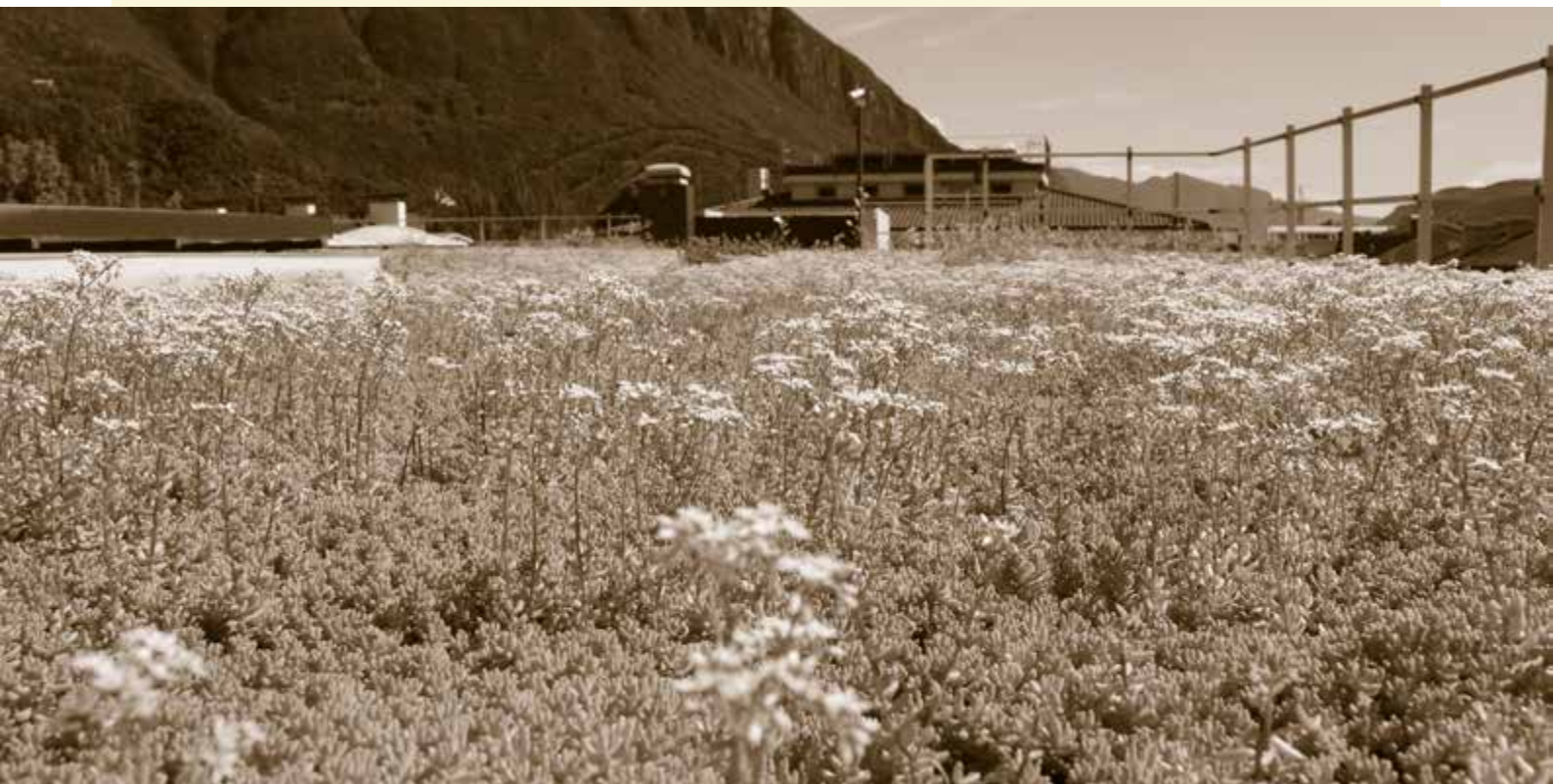
detail of the living roof of the Bolzano branch
